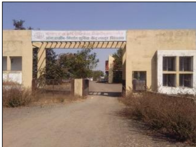
Export facility centre, Latur
