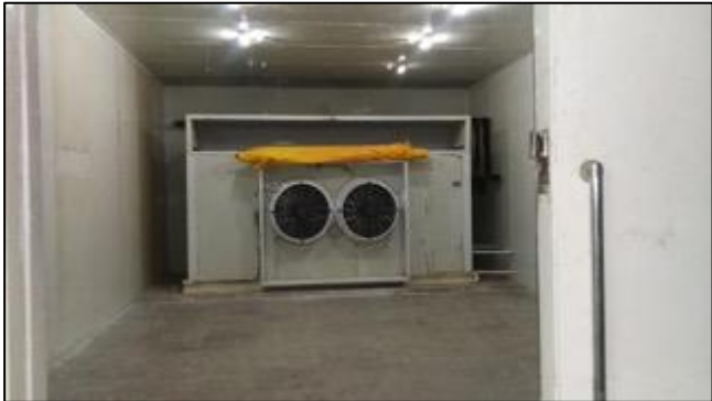
Pre cooling Export facility centre, Atpadi
