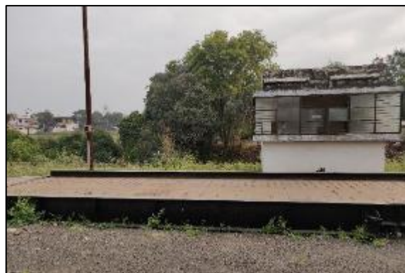
Weigh bridge, Export facility centre, Savda
