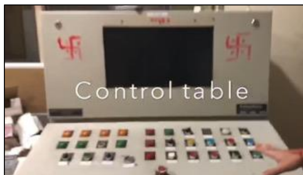
Control panel, Irradiation facility
