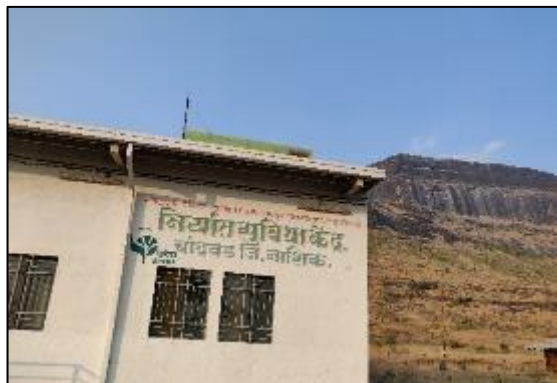
Chandwad Export facility
